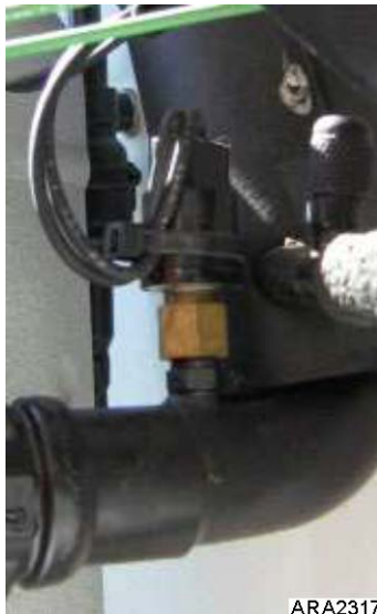
Low Pressure Cutout Switch Installed
