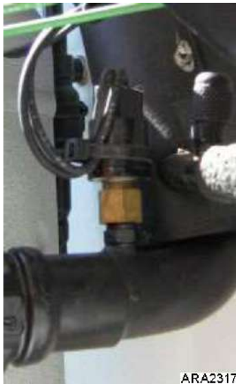
Low Pressure Cutout Switch Installed
