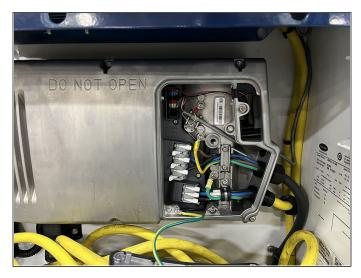
4. Release both sets of wires (compressor power cable and line power cable) from the VFD terminals. Make a note of the exact wire position as the same connections must be done on the replacement VFD.
