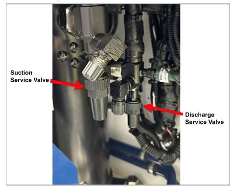
Figure 3.18 Compressor Service Valves
