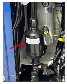
Figure 3.12 Filter Drier
