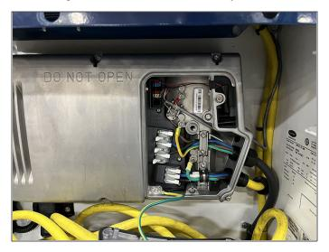
4. Remove and save the fan bolt by using a Torx T25 screwdriver. Then, loosen and pull out the fan wire grommet.
