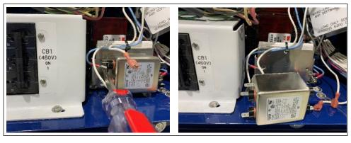
4. With the power filter removed, check for a capacitance reading of 0.54 uF +/-10% across pins 1 and 3. And then across pins 2-4.
