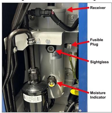
Figure 3.11 Receiver with Fusible Plug
