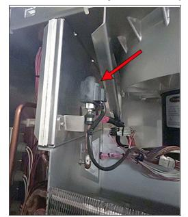
Figure 3.20 Electronic Expansion Valve (EEV)
