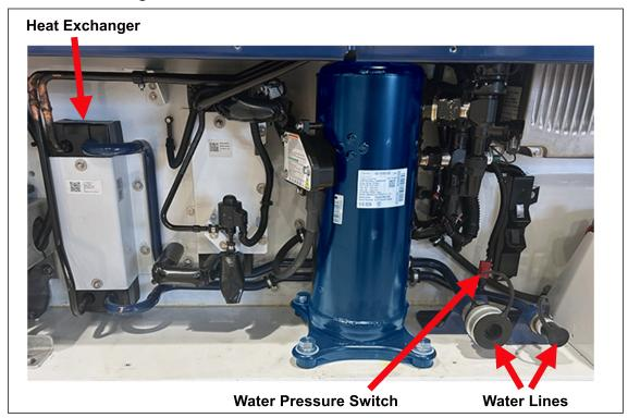
Figure 3.10 Brazed Plate Water-Cooled Condenser
