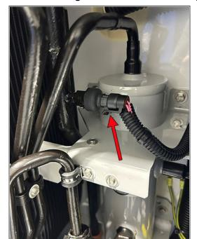
Figure 3.24 Discharge Pressure Transducer (DPT)
