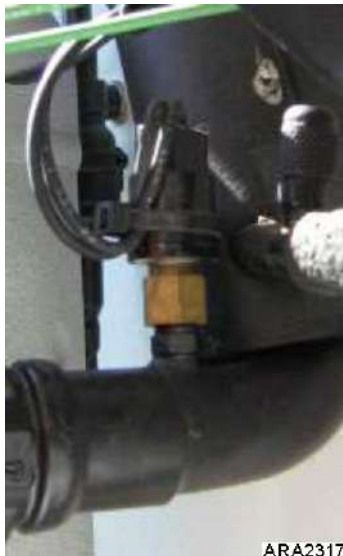
Low Pressure Cutout Switch Installed
